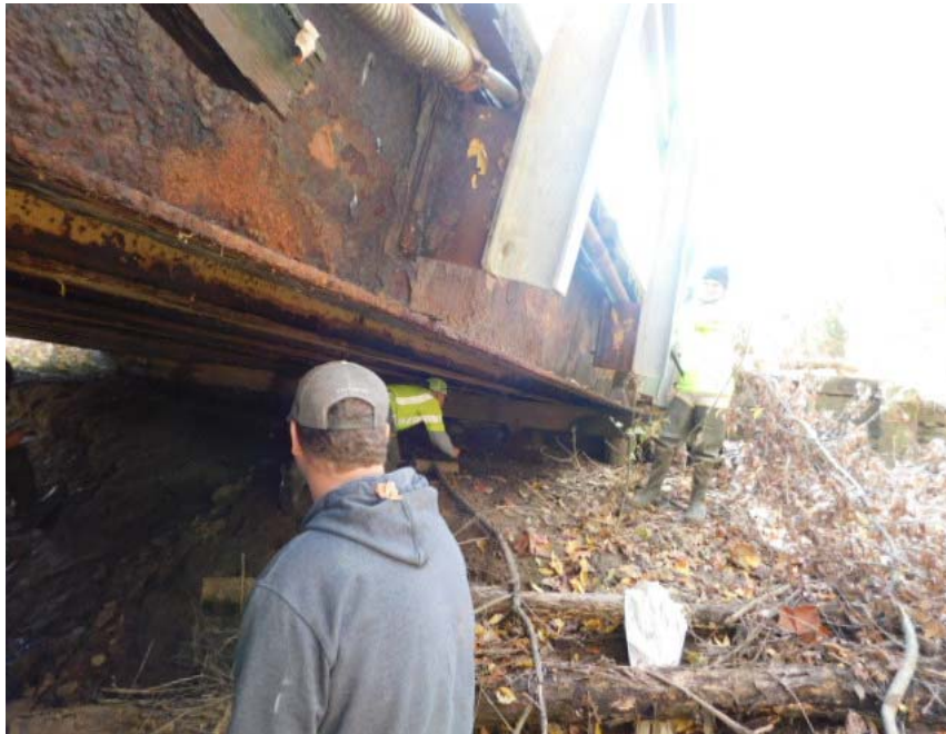
SPAN #1, STEEL "I" BEAM "A" WITH COLLISION DAMAGE
