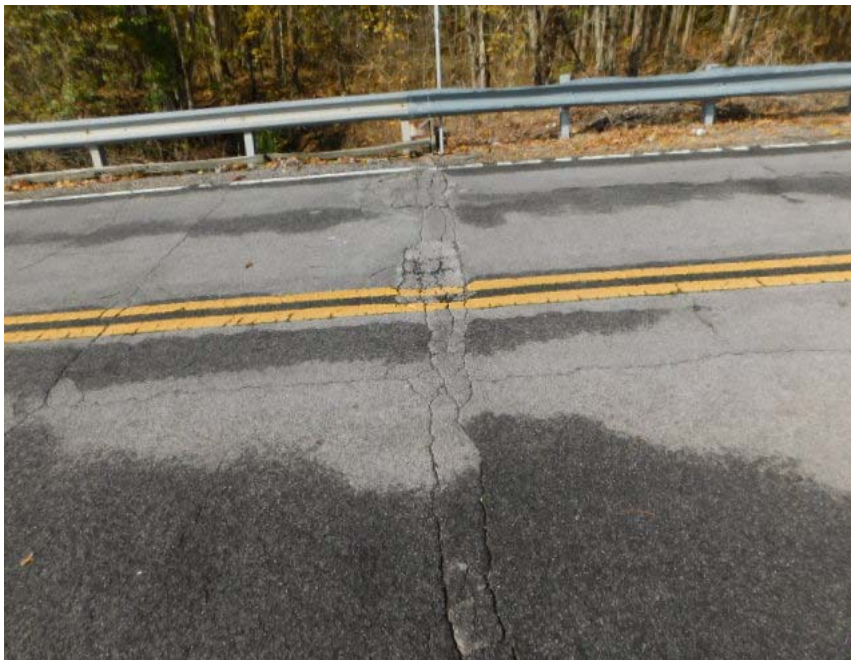
APPROACH #2 ASPHALT PATCHED & SETTLED
